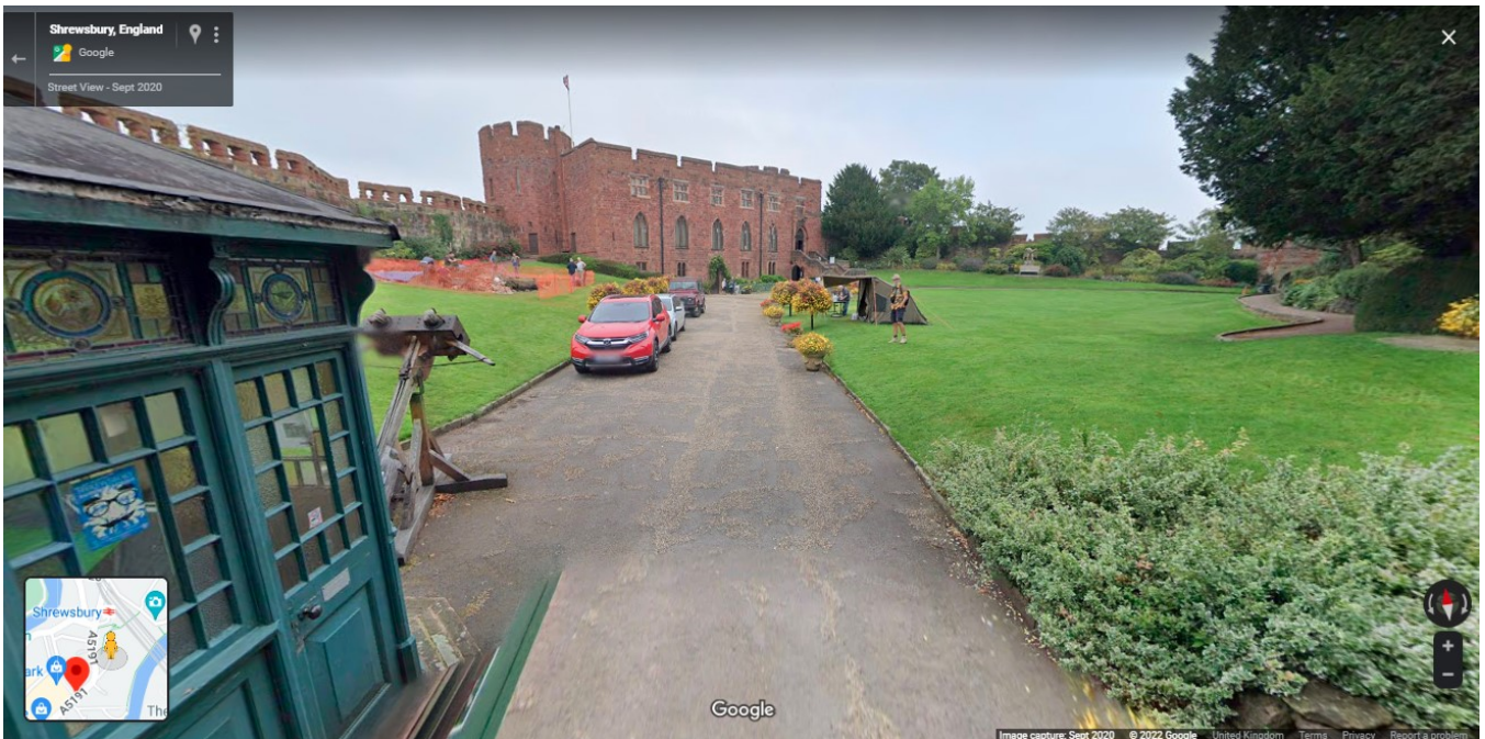
- View of the Castle from the main gates –
